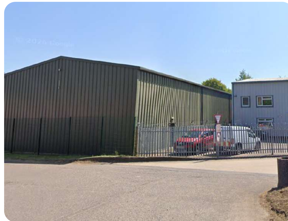
SHEPHERDS GROVE WEST INDUSTRIAL ESTATE LOOKING NORTH FROM READING LANE
