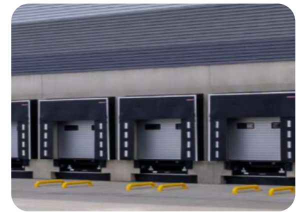
DOCK LEVELLER LOADING DOORS
