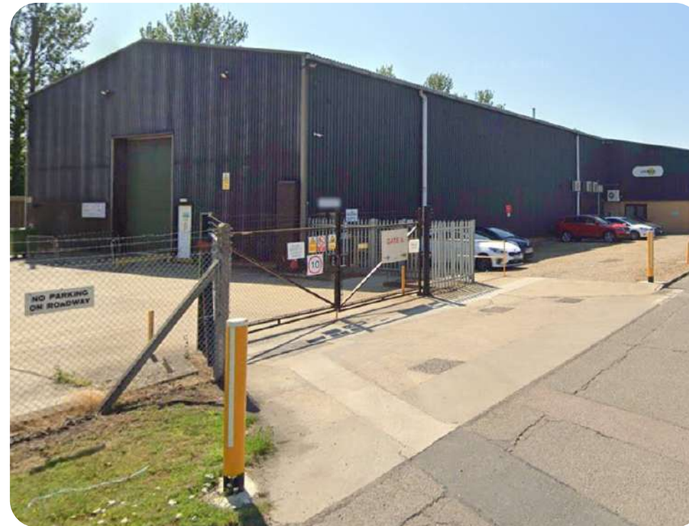
SHEPHERDS GROVE WEST INDUSTRIAL ESTATE LOOKING SOUTH EAST TOWARDS READING LANE
